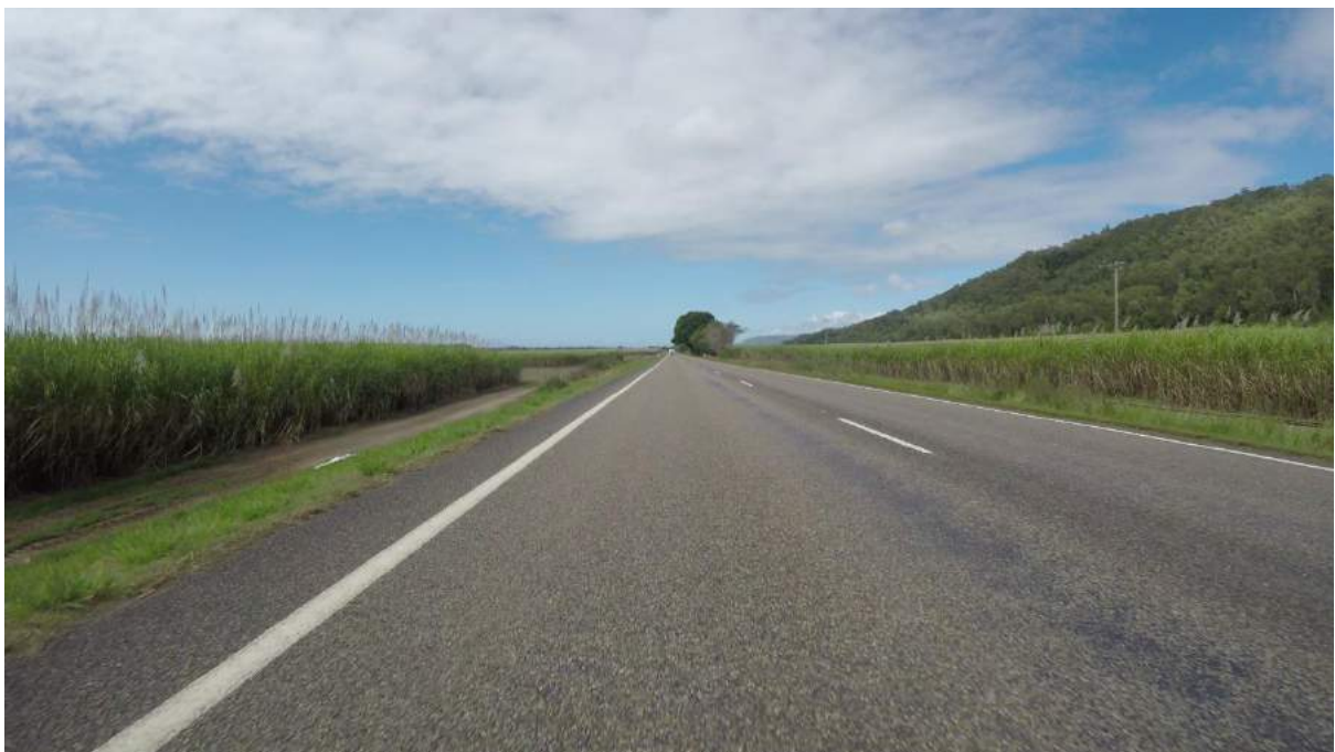
Flushing at 1400m
