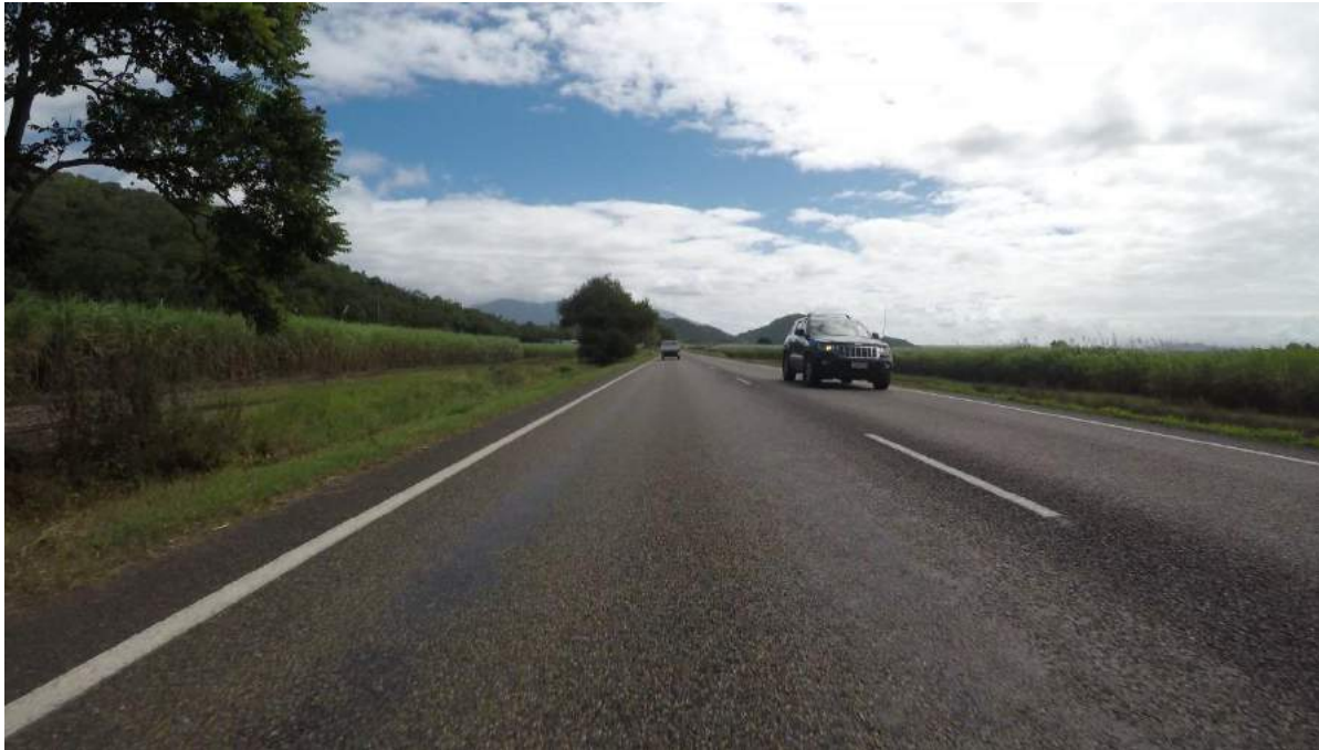
Flushing at 2100m
