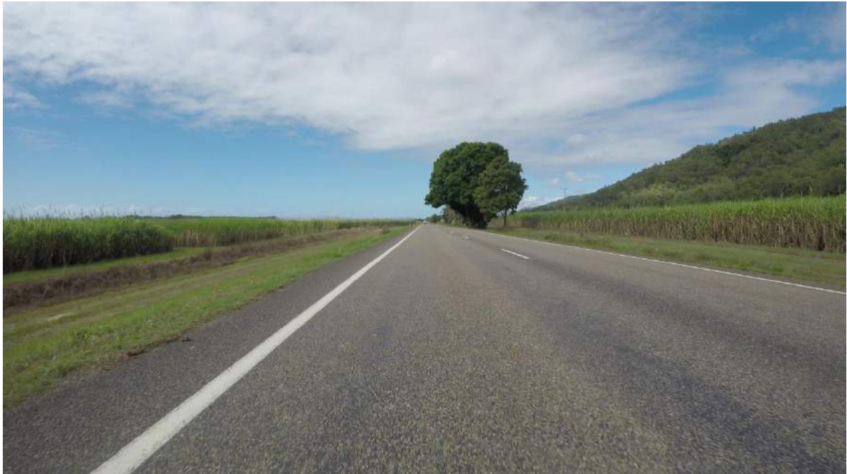
Flushing at 1600m
