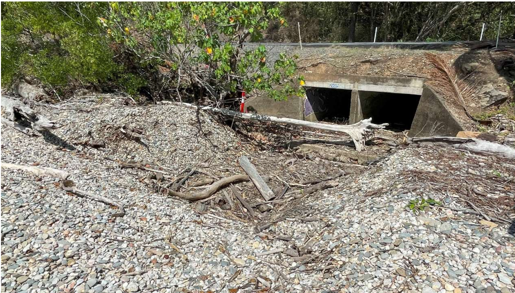
Figure 2-8: Existing culvert at site
