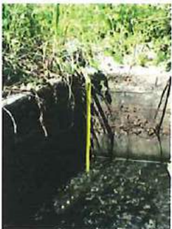
Plate 15. Standing water level east drain western end
