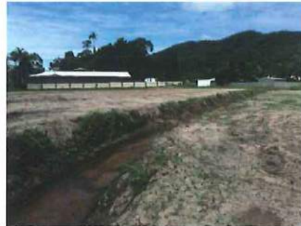
Plate 16. Southern drain near eastern boundary looking south west at recent drain works
