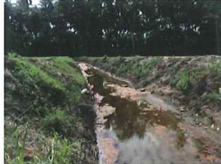
Plate 10. Mid-southern drain looking northeast
