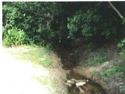
Plate 6. From Culvert at end of Marlin Drive looking west
