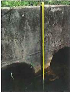
Plate 1. At northern drain culvert at Oasis drive
