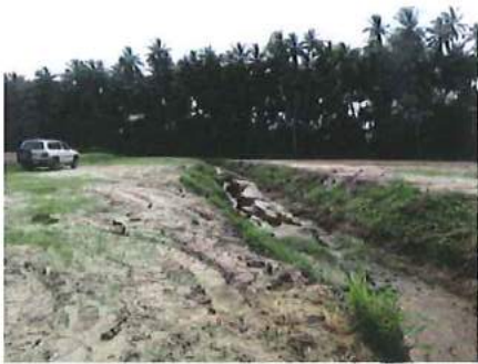
Plate 8. Central southern drain looking east at recent drain works
