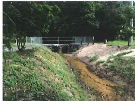
Plate 5. Southern drain looking west towards culvert at end of Marlin Drive
