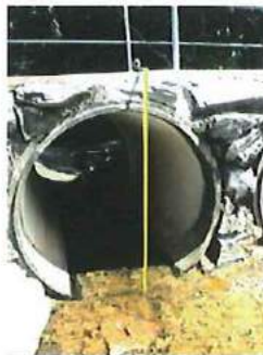
Plate 12. Standing water level southern drain at western boundary
