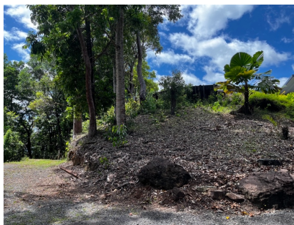
Image 3 – View of the existing vehicle track and erosion impact
