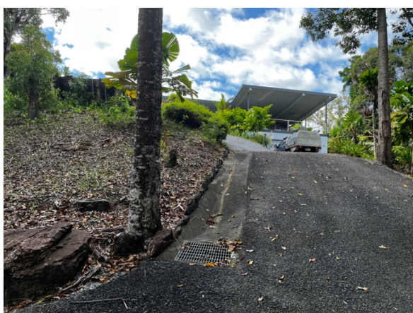
Image 2 – View of the existing driveway of the dwelling house
