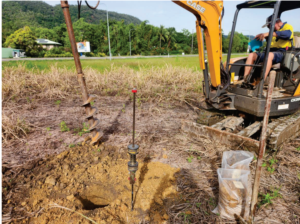
Site testing Andreassen Road Subdivision, Craiglie
