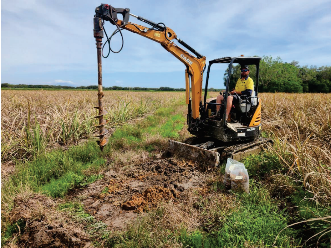
Site testing Andreassen Road Subdivision, Craiglie
