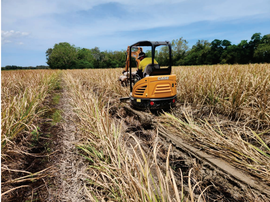
Site testing Andreassen Road Subdivision, Craiglie
