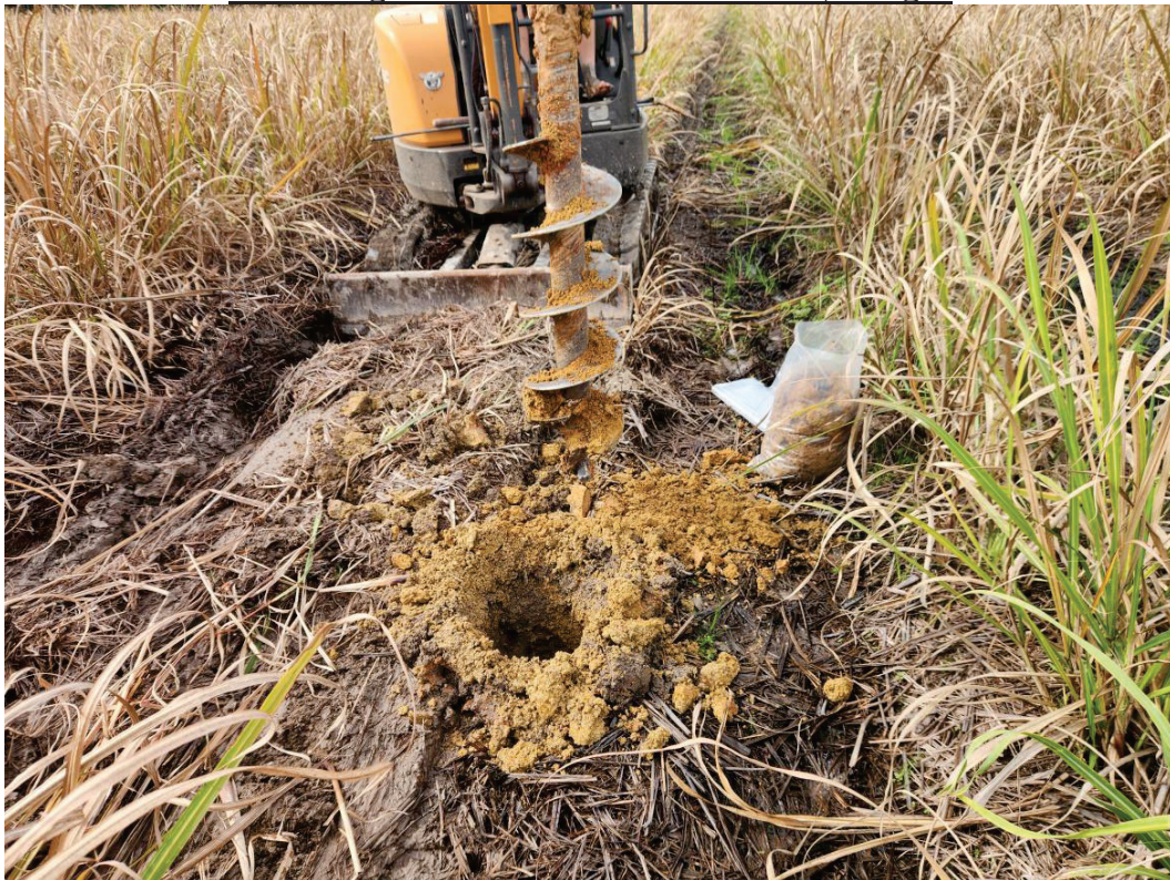
Site testing Andreassen Road Subdivision, Craiglie
