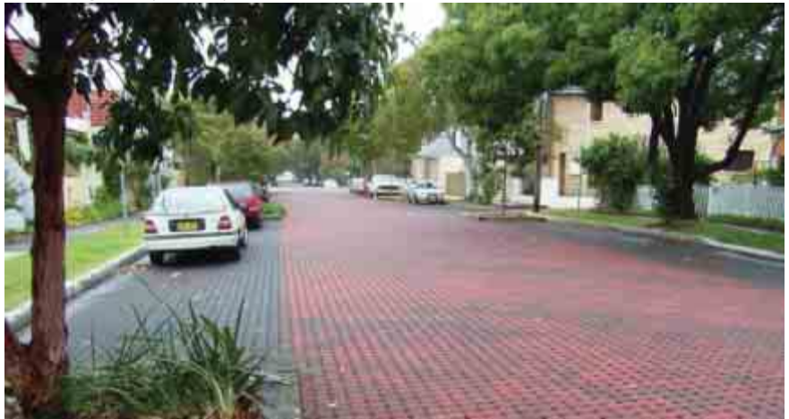
Interlocking block pavers - permeable road treatments for local streets or service access areas
