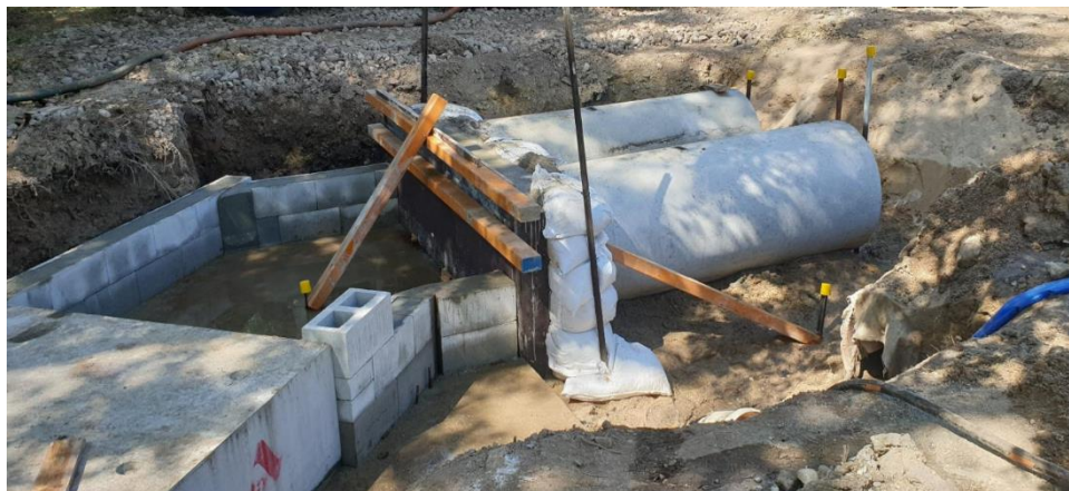
Image: Warner Street stormwater pit installation works
