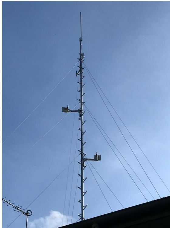
Image: One of nine transmitters installed around Port Douglas for the implementation phase 1 of the smart water meter project
