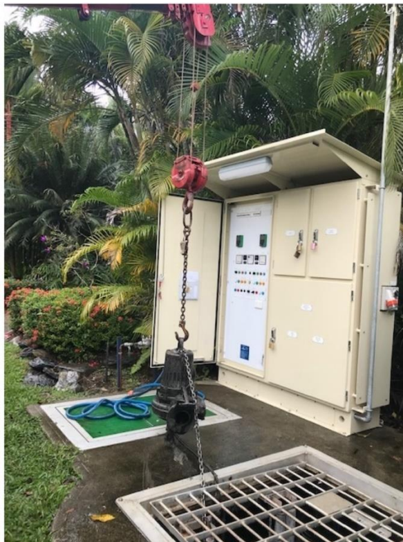
Image: Sewer pump station
