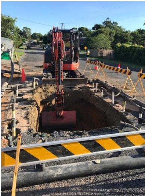
Images: Replacing a House Connection Branch at 11 Pringle Street, Mossman
