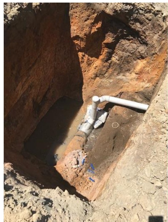
Images: Replacing a House Connection Branch at 11 Pringle Street, Mossman
