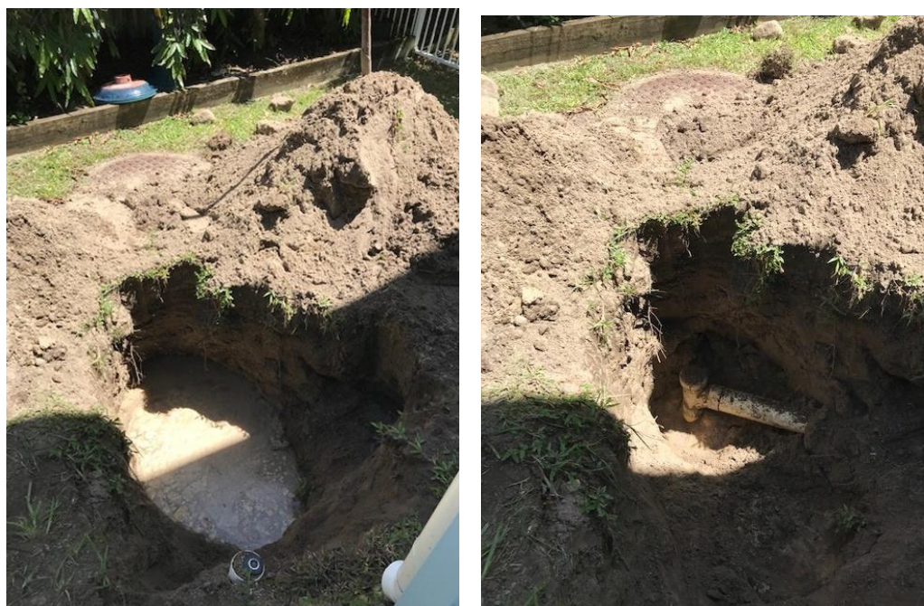
Images: Works carried out on a collapsed House Connection Branch on Andrews Close, Port Douglas
