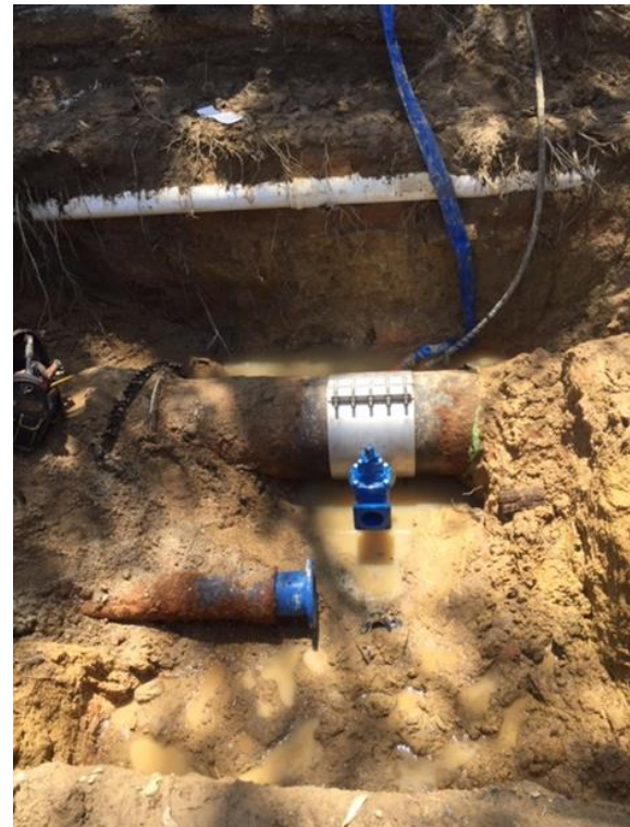
Images: Water Reticulation team replacing a faulty Wang Offtake Clamp and valve on the 450mm trunk main feeding Port Douglas reservoirs, located at the corner of Coral Sea Drive, Mossman
