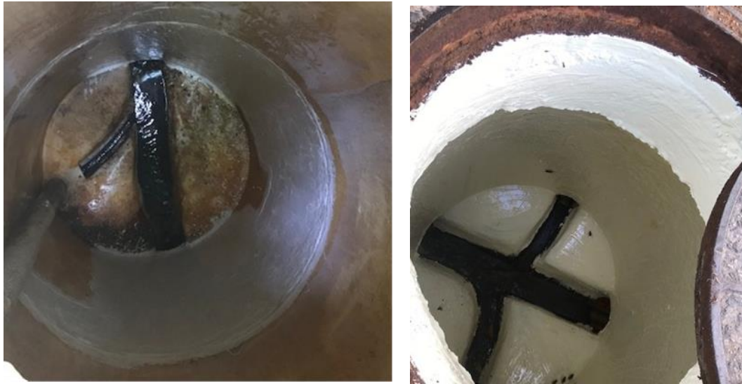
Images: Wastewater Manhole Raising Project, showing a deteriorated manhole on the left and a refurbished manhole on the right
