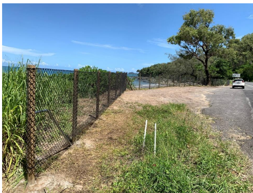
Image: Fence installed at Borderline Beach to restrict vehicles driving along the beach
