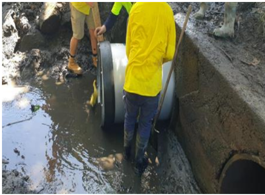
Image: Tide gate installed at Mudlo Street
