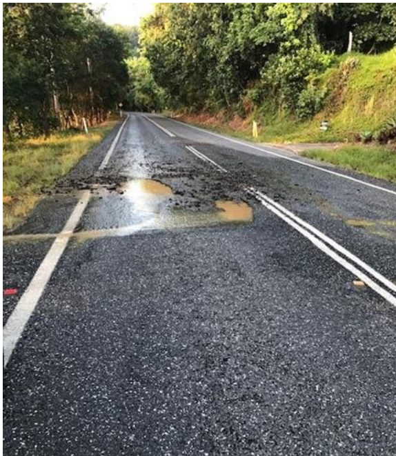
Images: Water Reticulation team responding to a water main break between Rocky Point and Wonga Beach
