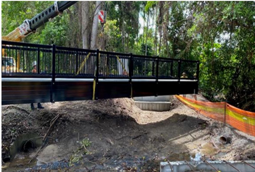
Image: Lowering of the pedestrian bridge into position
