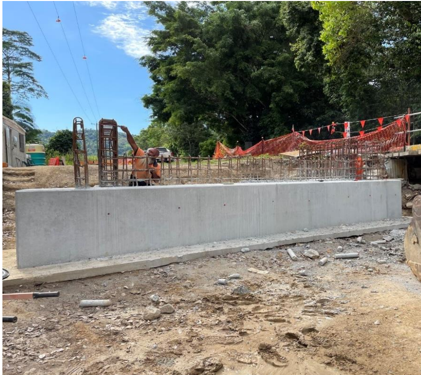
Image: Warner Bridge Abutment Construction
