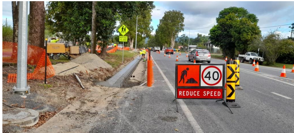
Images: New section of Kerb and Channel renewal in Alchera Drive, Mossman
