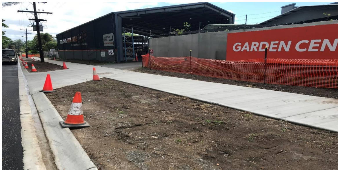
Image: New section of Kerb and Channel renewal in Mossman St, Mossman
