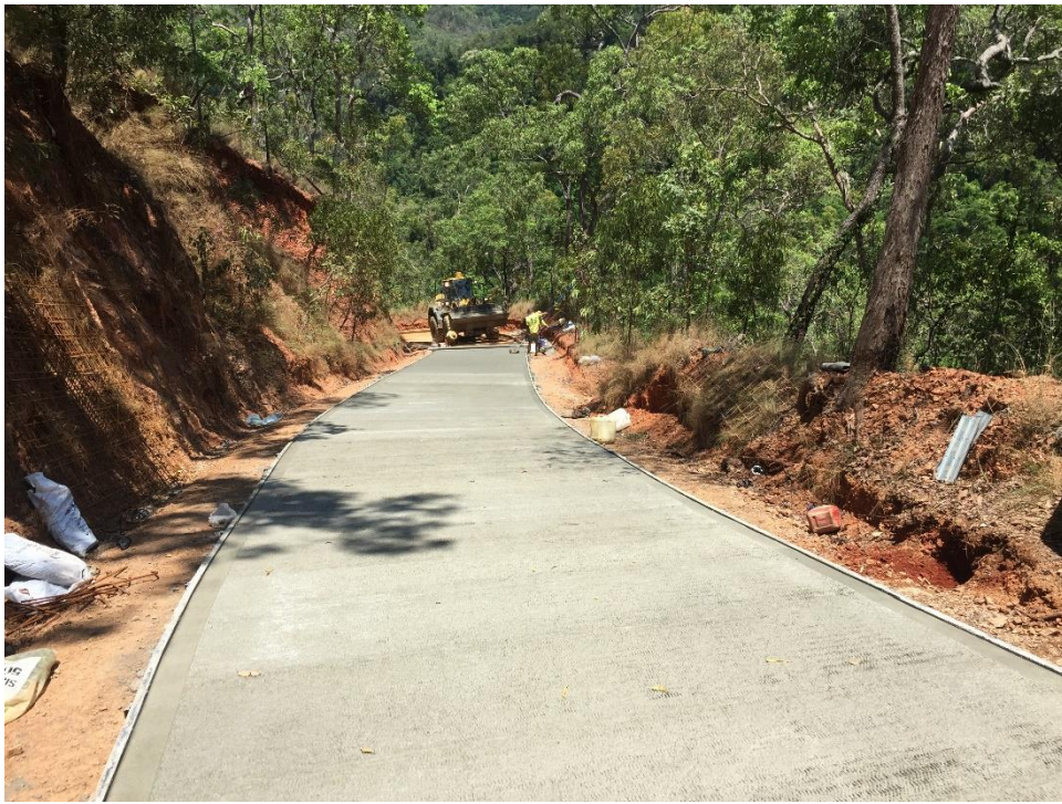
Image: New concrete pavement being installed on Zig Zag Road, Degarra
