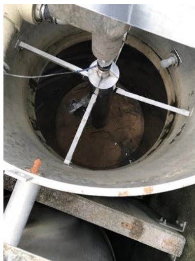
Images: Replacing backwash filter sand at the Port Douglas WWTP Ordinary Council Meeting - 25 January 2022
