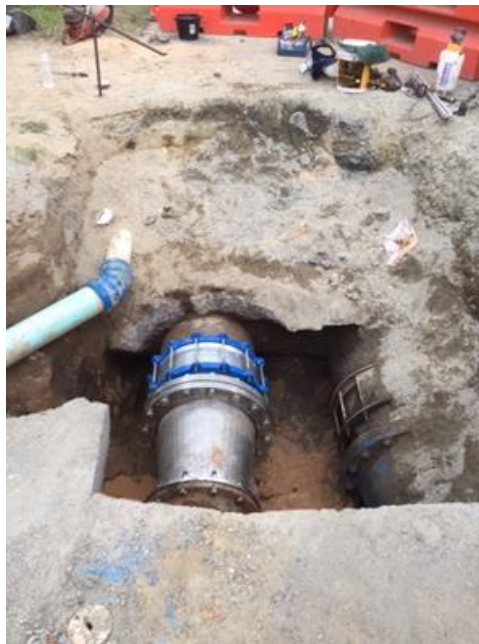
Image: Work being undertaken on the treated water main on Coral Sea Drive. These parts had to be manufactured by a local engineering company due to the unavailability of standard fittings.
