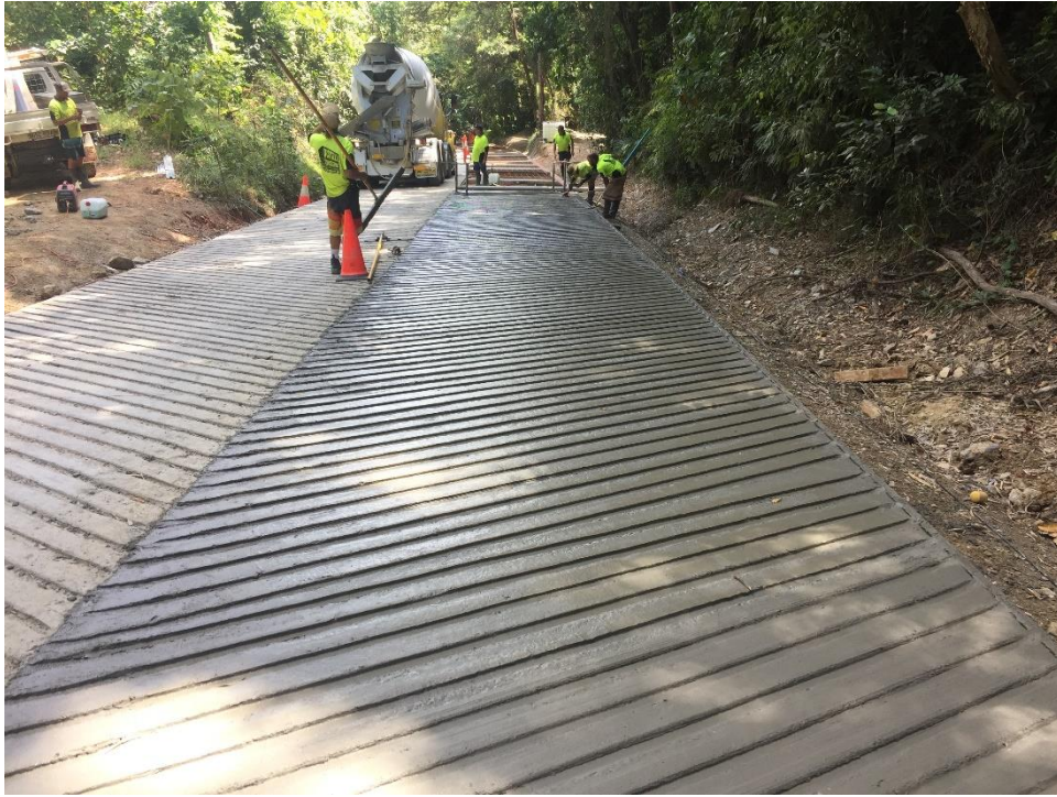
Image: New concrete pavement on Cape Tribulation Bloomfield Road at Donovan's Range being installed
