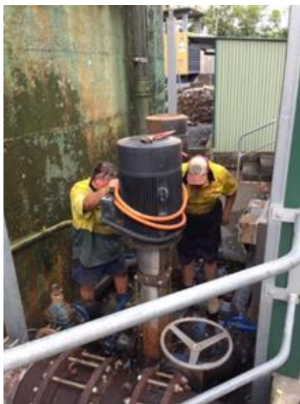
Images: Redundant pumps and equipment removal at Mossman WTP
