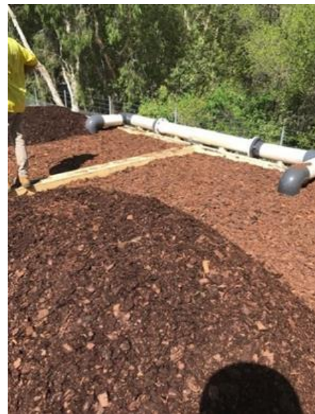
Images: Refurbishment of the odour control unit
