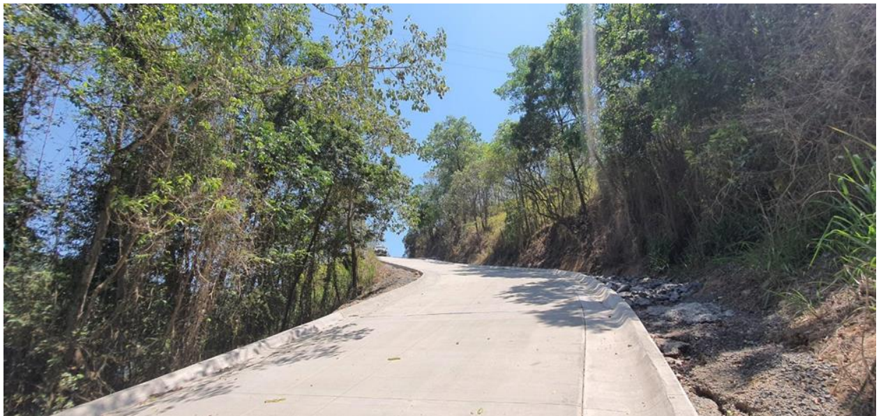
Image: New concrete pavement on steep section of Cape Tribulation Bloomfield Road known as Pierces Hill
