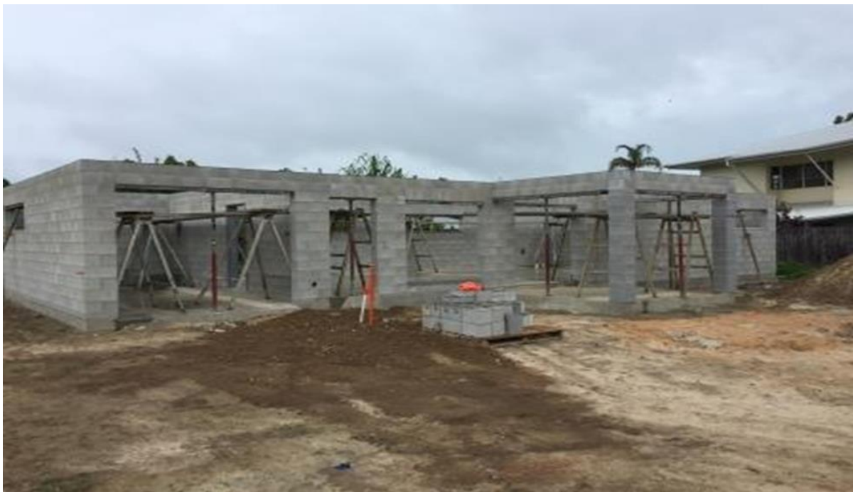
Image: Blockwork erected
