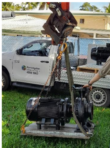
Images: Installation of new water pump at Mossman Pool
