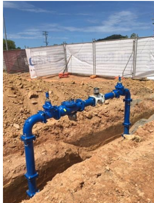
Images: Water Reticulation team and local plumbers working together to install a new water service for the Mossman Fire Station
