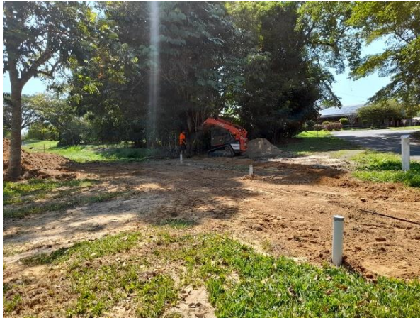
Images: Installation of new toilet dispersal area
