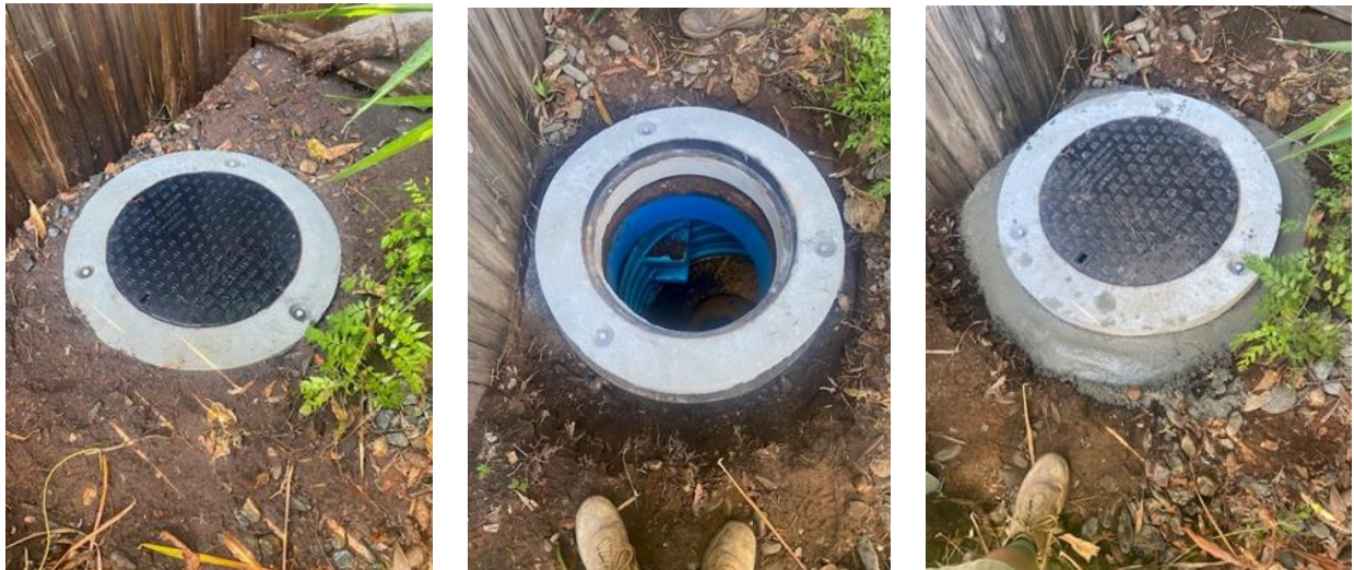
Images: Wastewater Manhole Raising Project, showing a manhole that has been raised
