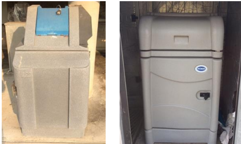
Images: Replacement auto sampler (right) at Mossman WWTP
