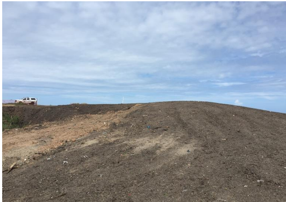
Image: Killaloe Landfill closed, rolled and seeded
