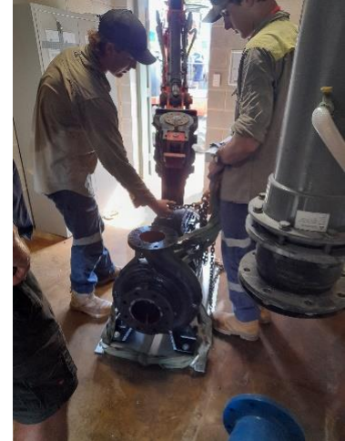
Images: Installation of new water pump at Mossman Pool
