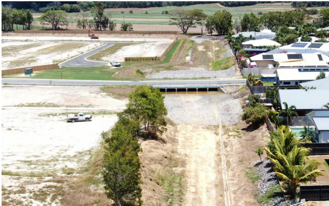
Image: Cleaning out stormwater drainage in preparation for the wet season
