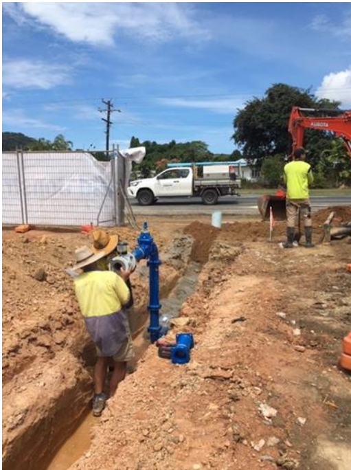
Images: Water Reticulation team and local plumbers working together to install a new water service for the Mossman Fire Station
