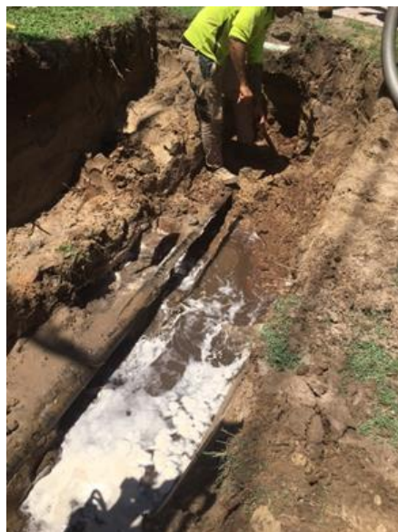
Images: Water Reticulation team fixing a main break in Seabrook Avenue, Port Douglas. Six metres of pipe was replaced
