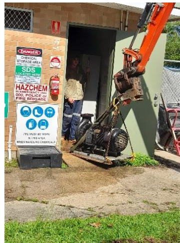
Images: Installation of new water pump at Mossman Pool
