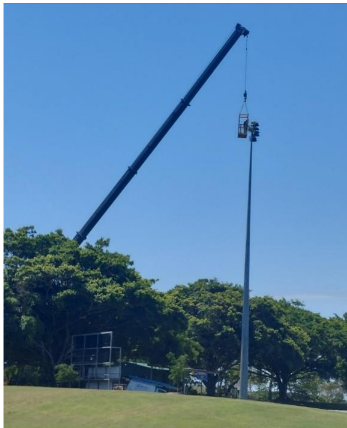
Image: Port Sports Complex – Light globes and ignitors being replaced
