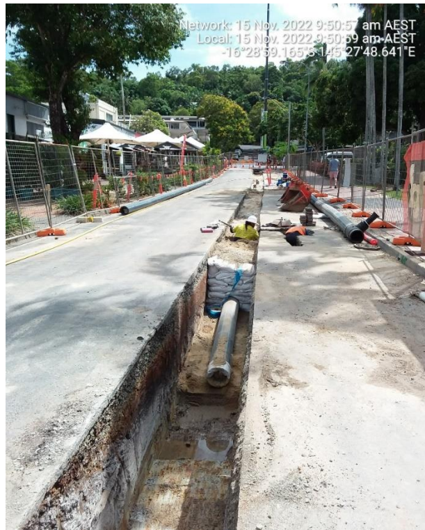
Image: Water main being laid Grant St, Port Douglas
