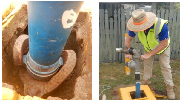
Image of standpipe on base, between the locating hooks and turning standpipe clockwise
