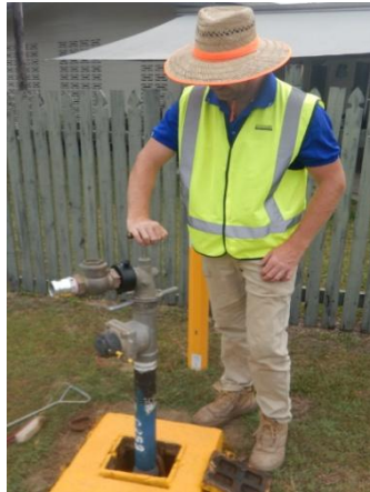
Image of turning Tee Top anticlockwise
