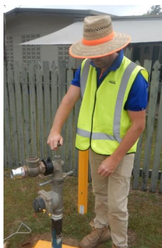
Image of turning the Tee Top clockwise to allow water extraction
