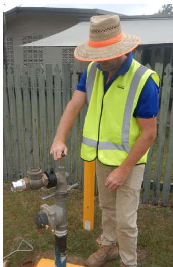
Image of turning the Tee Top clockwise to allow water extraction
