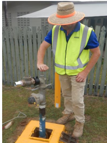
Image of turning Tee Top anticlockwise
